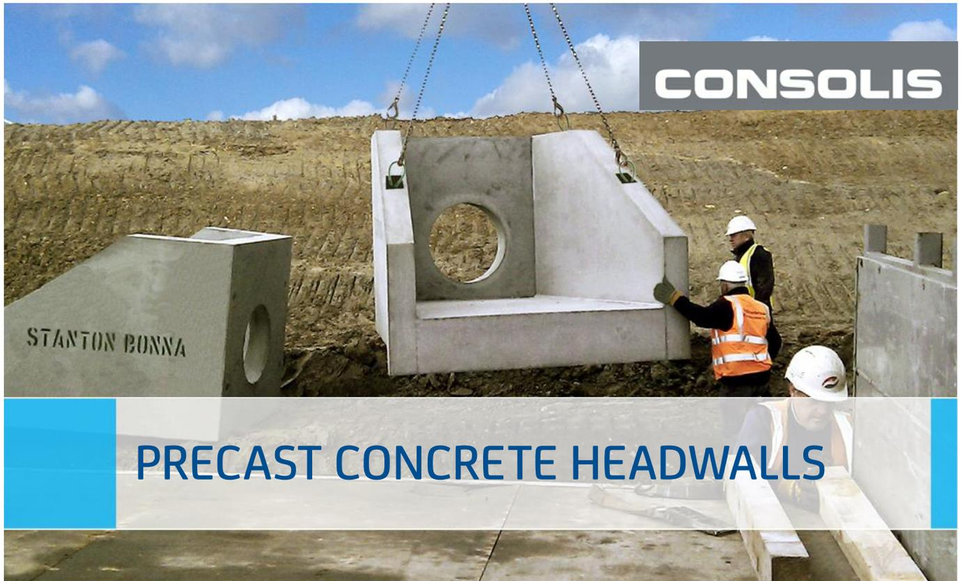
Precast concrete headwalls for drainage outfall connections into open water areas including collection ponds, swales and rivers.
