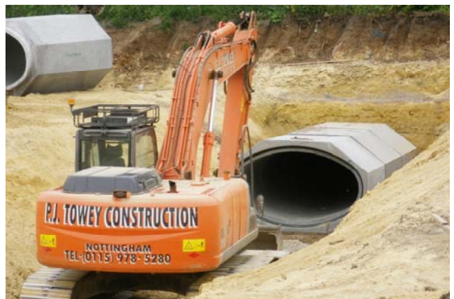
The pipeline installation was at a low cover level so strength of the system was as important as efficient flow
