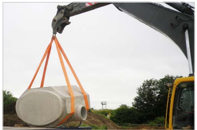
Elliptical pipe with end wall and 600mm diameter spigot
